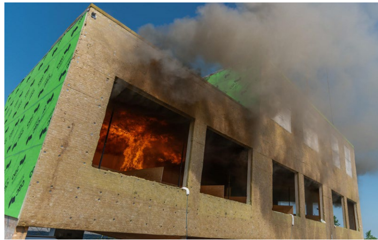
Image: Fire developing within mass timber structure.
