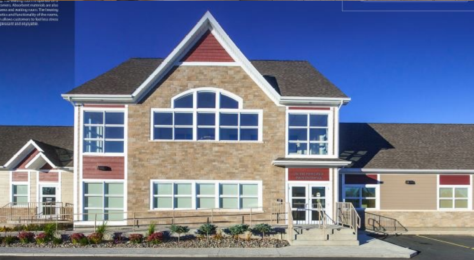
E. Arseneau Audiology Clinic Clinique D'Audiologie E. Arseneau Aedifex Architecture Inc. (Currently CLAD Inc.)
